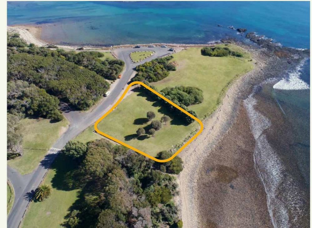
Aerial view of the proposed site at Don Head Foreshore
